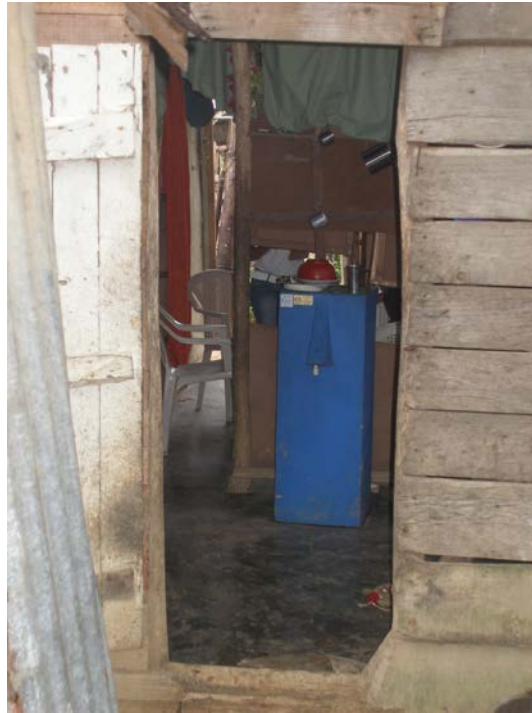
Figure 2.2 – Biosand filter in Dominican Republic home
