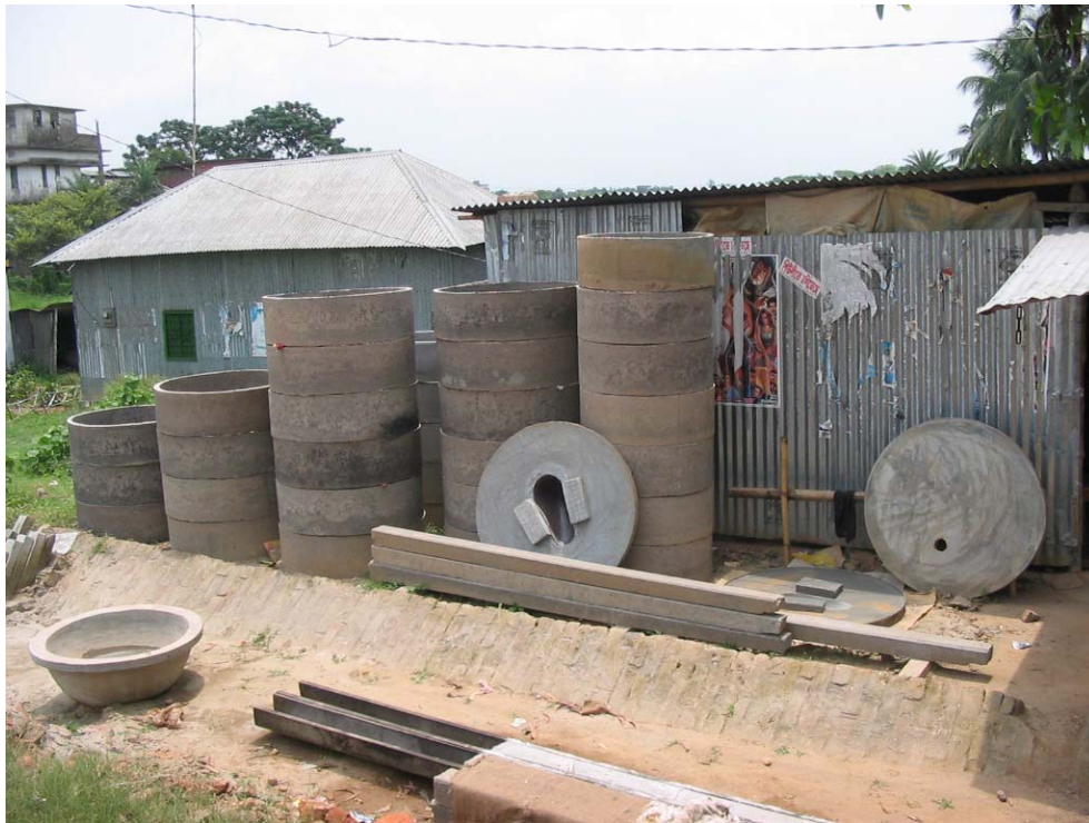
Factory for manufacturing concrete rings and bases for latrines, wells and water storage tanks.
